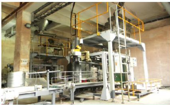
CHEMICAL PACKING MACHINE LINE
