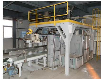
CHEMICAL PACKING MACHINE LINE
